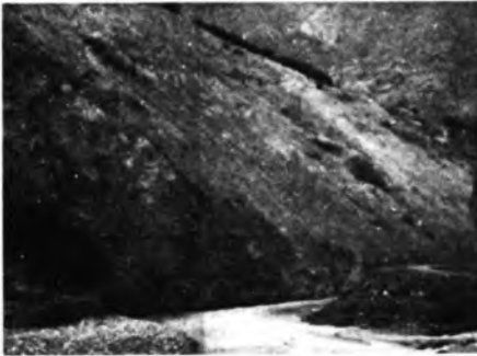
Fig. 5: Havuzlu landslide view from upstream
