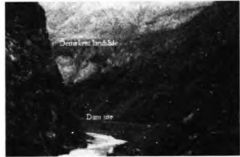
Fig. 6: Inanli dam site and Demirkent landslide view from upstream
